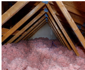
Fiberglass Blown – R-2.8 / inch
