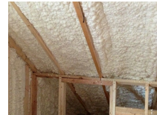
Closed Cell Polyurethane – R- 6.0 / inch
