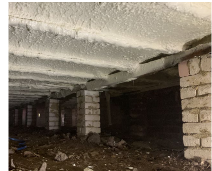
Closed Cell Polyurethane – R- 6.0 / inch
