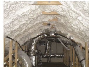
Open Cell Polyurethane – R- 3.7 / inch
