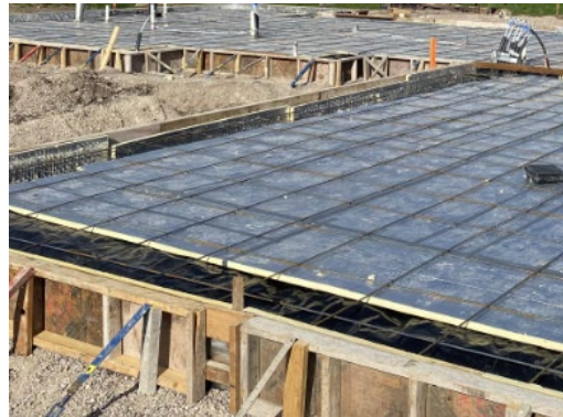
Polyisocyanurate Board – R-7 / inch
