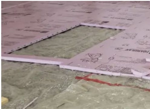
Extruded Polystyrene Board – R-5 / inch
