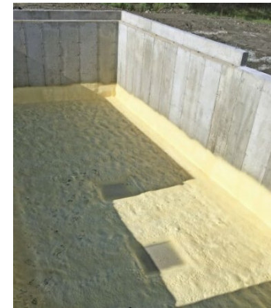
Closed Cell Polyurethane – R- 6 / inch
