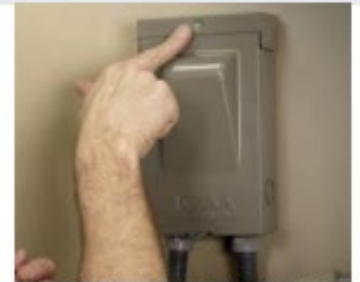
Figure 2: Integrated electrical disconnect with surge protector
