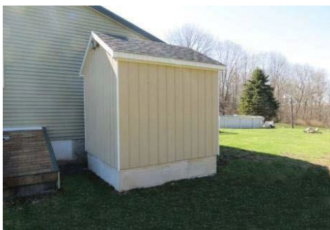
This 4.5-ton outside residential bulk wood pellet storage bin has a ventilated soffit and two ports for pellet delivery
