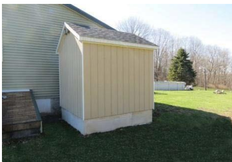
This 4.5-ton outside residential bulk wood pellet storage bin has a ventilated soffit and two ports for pellet delivery
