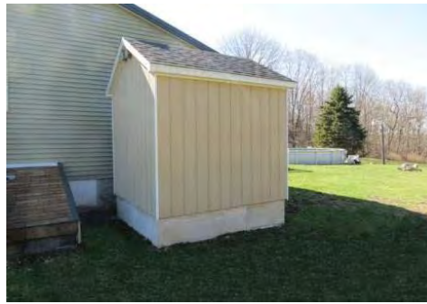
Figure 1. This 4.5-ton outside residential bulk wood pellet storage bin has a ventilated soffit and two ports for pellet delivery. (Photo courtesy of Vincent’s Heating and Fuel Service LLC)
