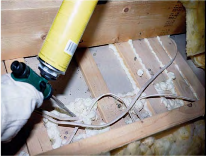
Top Plates Sealed with 1-Part Foam ( Click to Return to Section )
