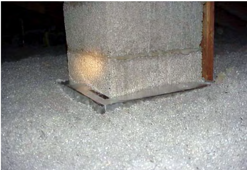
Attic Insulation Dammed Away from Chimney ( Click to Return to Section )
