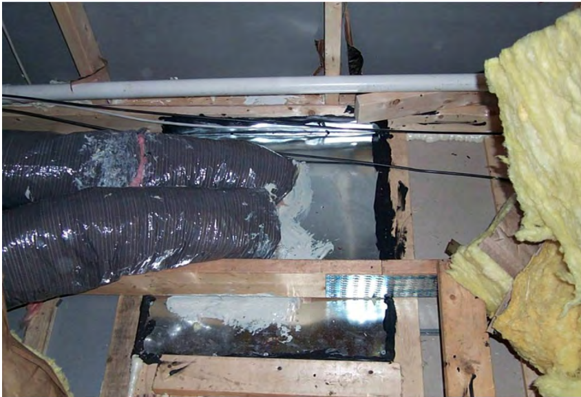
Open Attic Chase Sealed with Sheet Metal, Duct Mastic and Acoustical Sealant ( Click to Return to Section )
