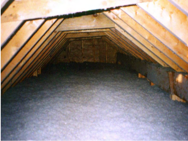
Loose Fill Attic Insulation Evenly Installed ( Click to Return to Section )
