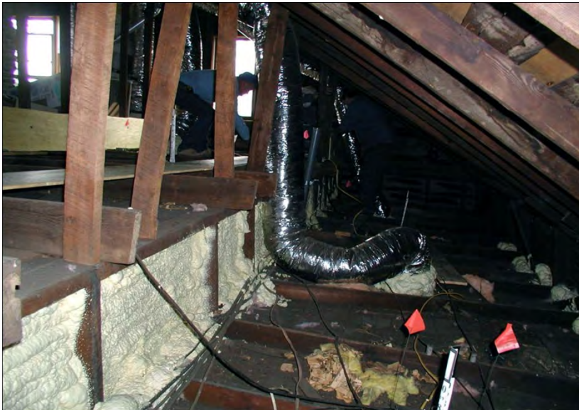
Ceiling Height Transition Wall Sealed with 2-Part Foam ( Click to Return to Section )
