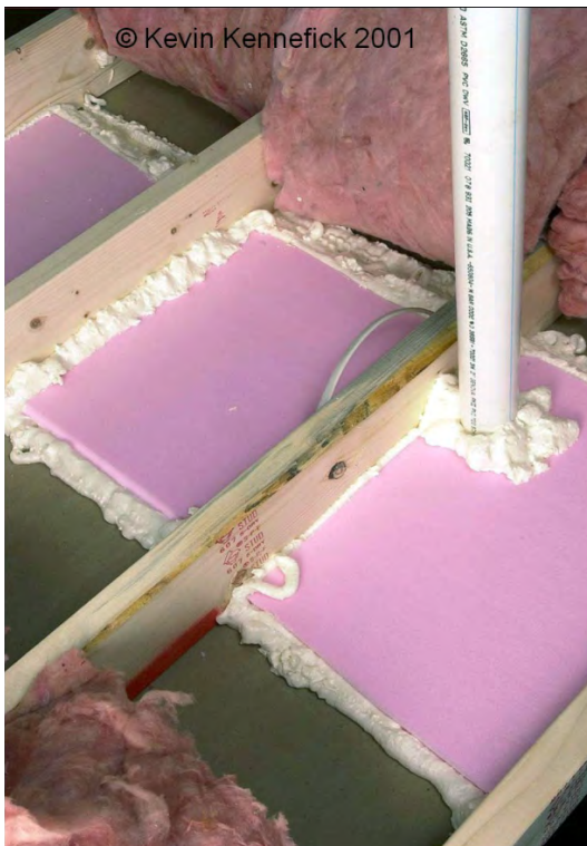
Dropped Soffit Sealed with XPS and 1-Part Foam ( Click to Return to Section )
