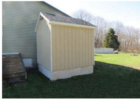
Figure 1. This 4.5-ton outside residential bulk wood pellet storage bin has a ventilated soffit and two ports for pellet delivery.
