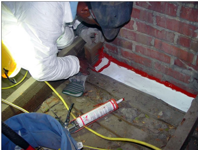
Chimney in Attic Sealed with High-Temp Caulk and Metal Flashing ( Click to Return to Section )
