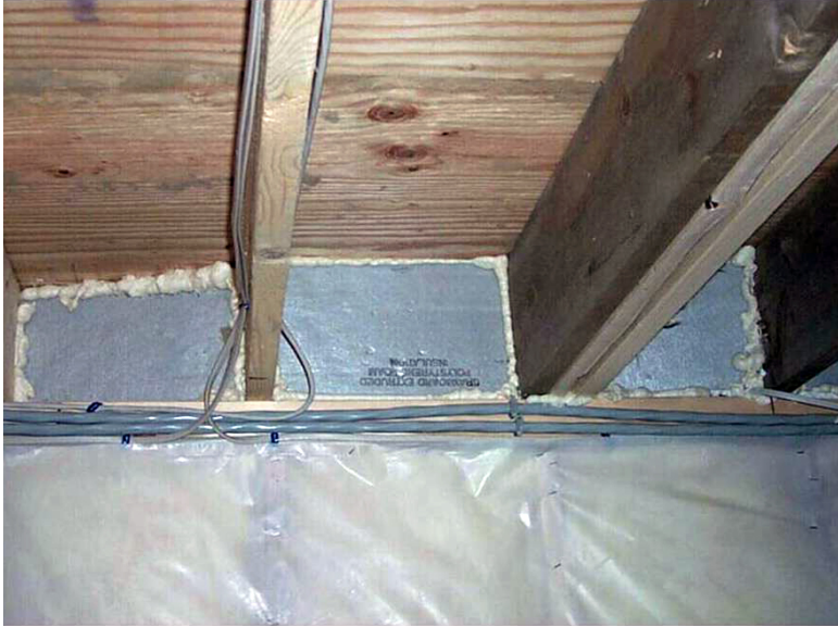
Rim Joist Insulated (and Sealed to Sill) with Foam Board and 1-Part Foam ( Click to Return to Section )
