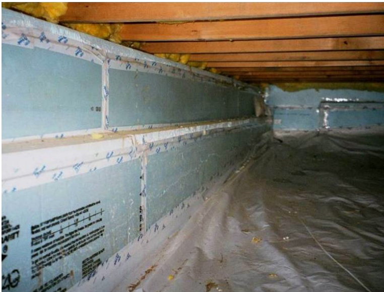
Crawlspace Ground Cover ( Click to Return to Section )
