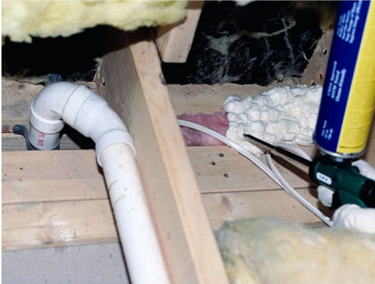
Plumbing Wet Wall Sealed with Fiberglass Batt Backer and 1-Part Foam ( Click to Return to Section )
