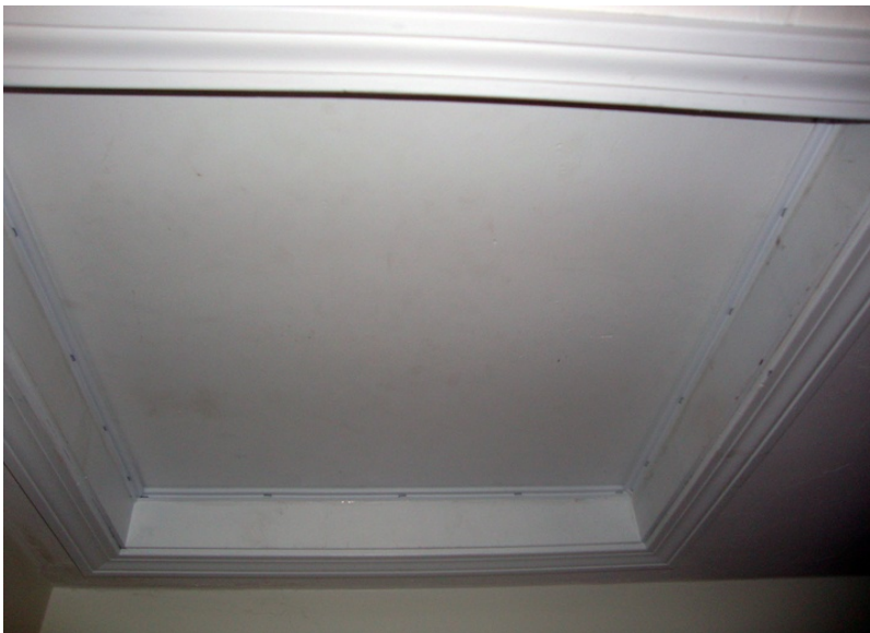
Attic Hatch Weather-stripped ( Click to Return to Section )
