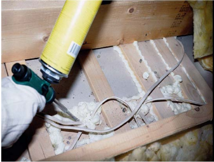
Top Plates Sealed with 1-Part Foam ( Click to Return to Section )
