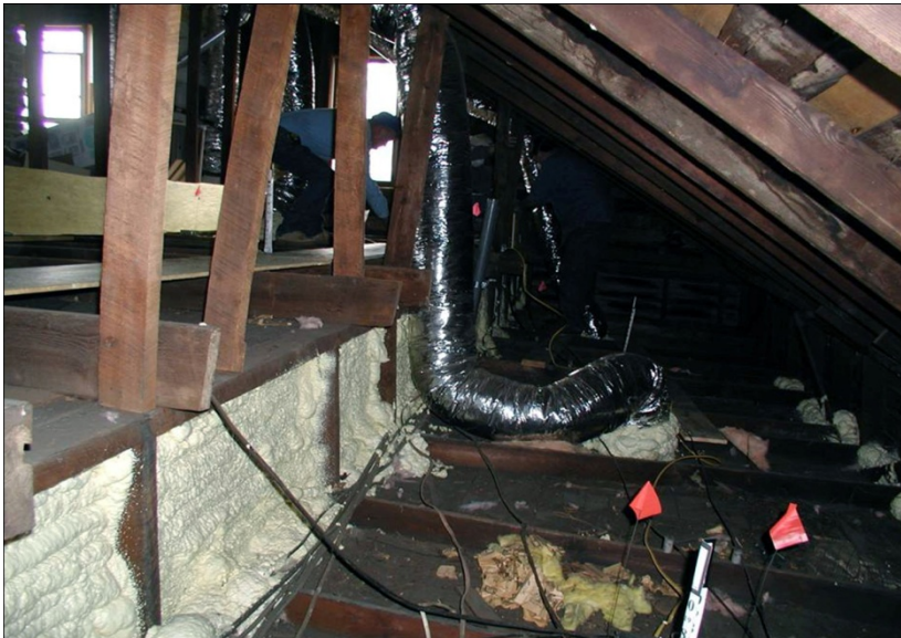
Ceiling Height Transition Wall Sealed with 2-Part Foam ( Click to Return to Section )
