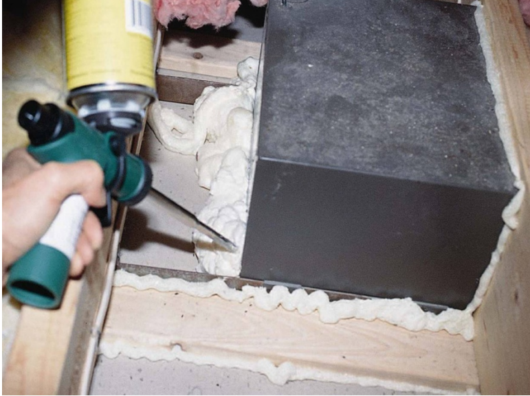
Bath Fan Sealed with 1-Part Foam ( Click to Return to Section )
